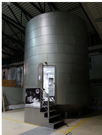
Figure 5: Photo of the mock-up exterior. The two-story mock-up is constructed from wood and dry wall and located inside Hall 2 of the ZARM.
