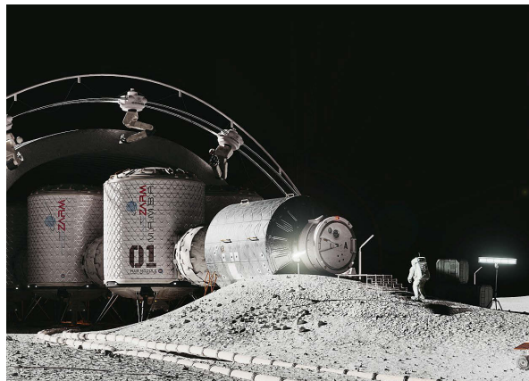
Figure 1: Artistic rendering of a habitat based on the MaMBA concept. One can see two of the main modules, one airlock and two of the inflatable connecting modules. The radiation shield is under construction in this image.
